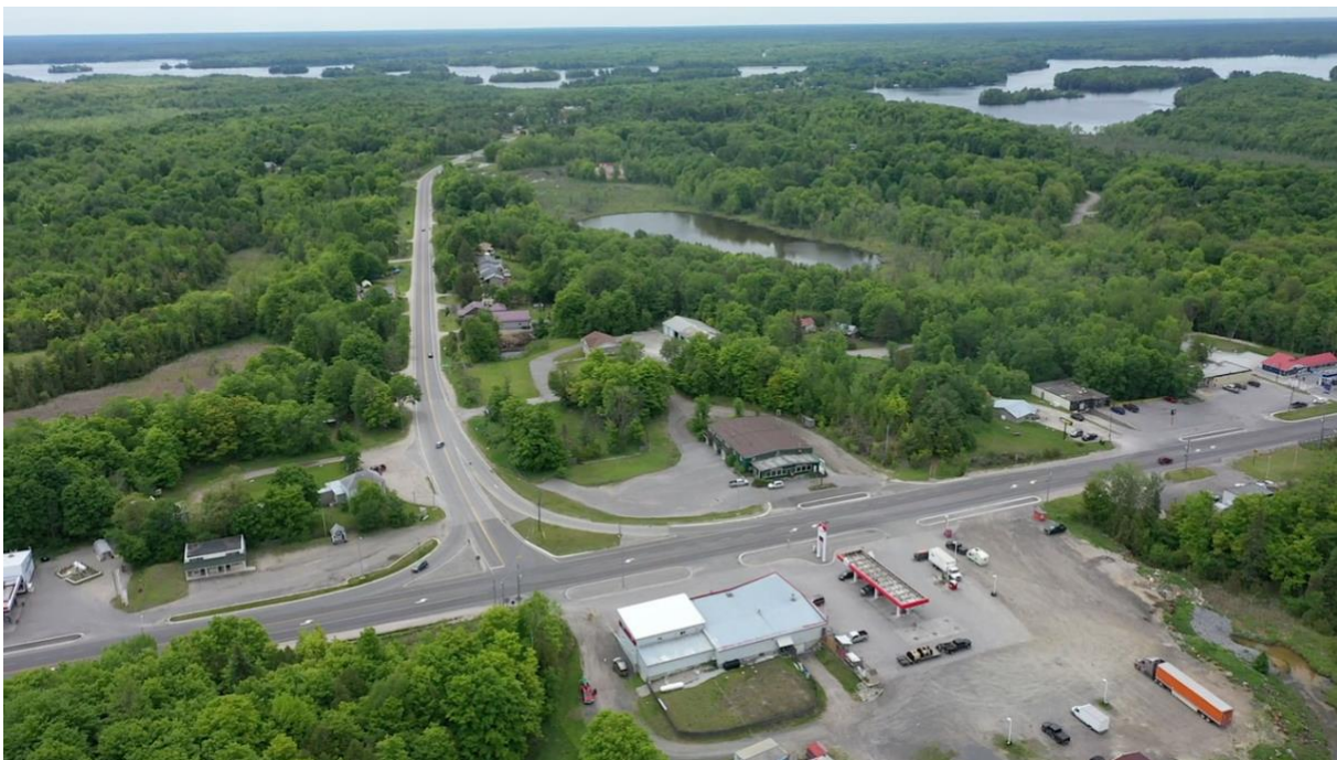
Intersection of Road 38 with Highway 7 as seen from the north. (Wade Leonard – Above & Beyond)
