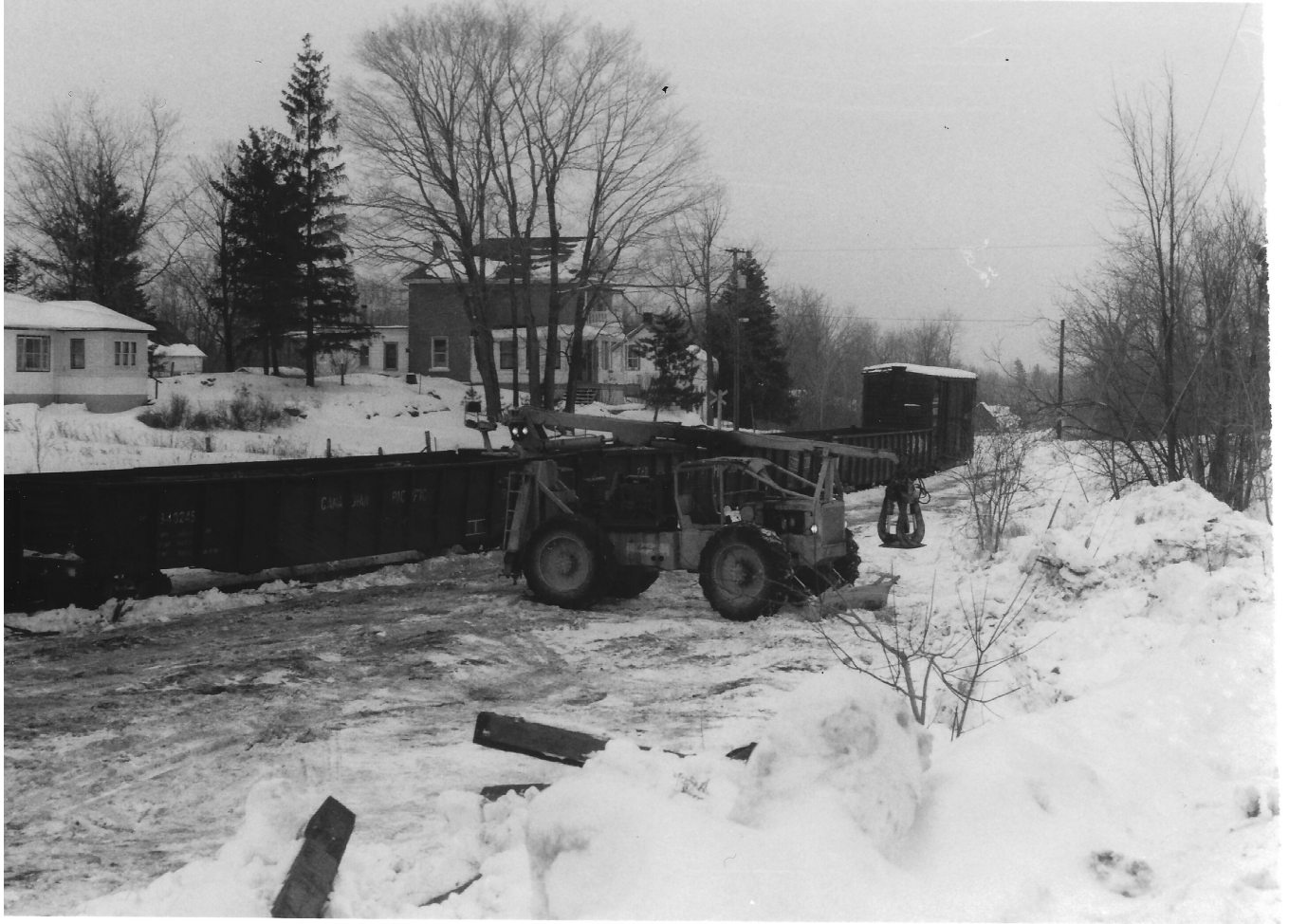
The K&P Siding Yard at Tichborne, looking south. The tall crane with the electromagnet was loading rail into the gondolas. The rails between Verona and the Tichborne yard were hauled in by road trucks.
