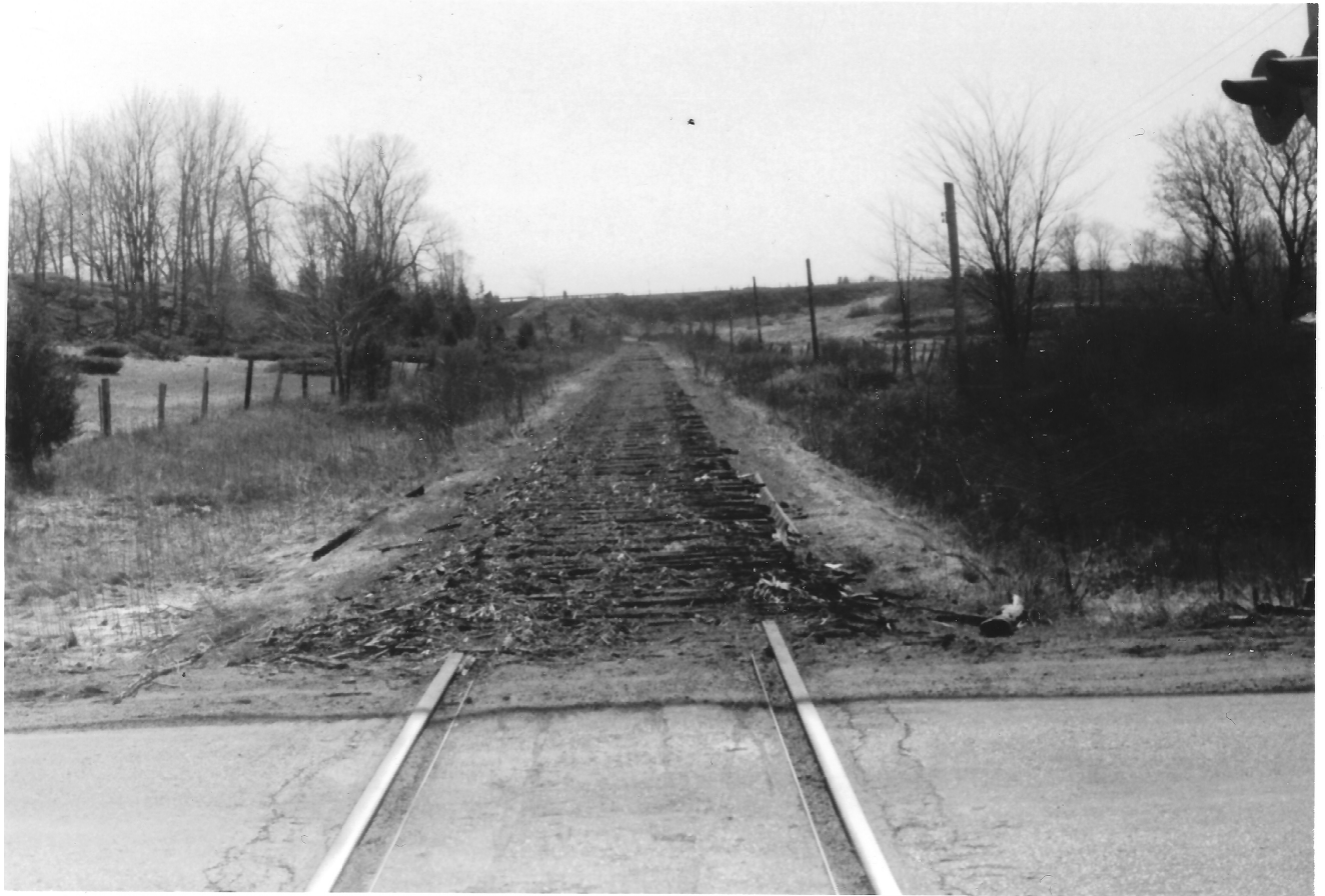
The rail line looking north from the Fifth Concession Road crossing at Jackson's Mills. The track curve in to the large horseshoe bend around to the left. The ties along this part of track were taken up and plied on April 10 th .
