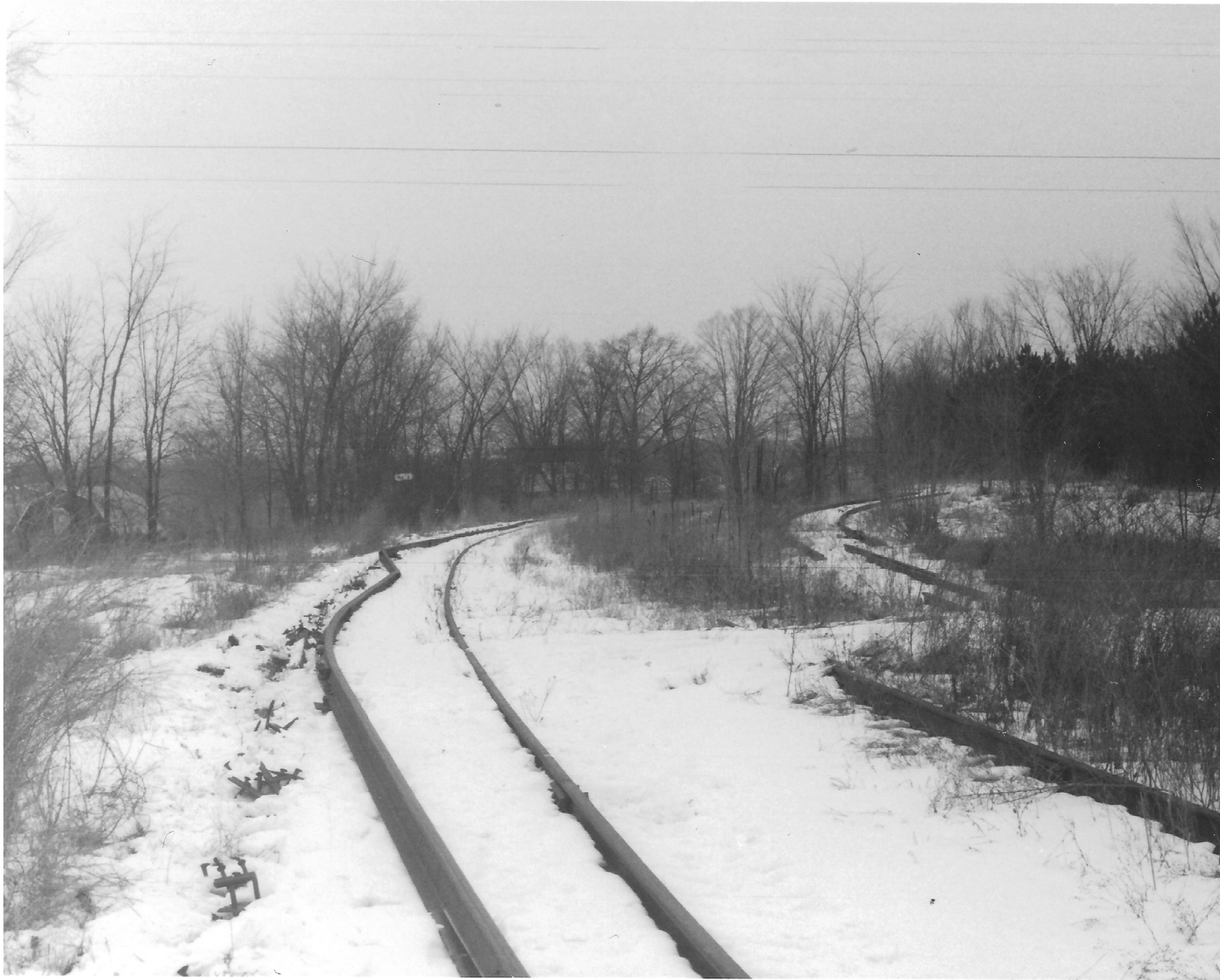
The rail line at Murvale Station site looking north. The west (left) rail has been lifted. At the left is the trolley shed. The siding swings in to the right from the south end switch.
