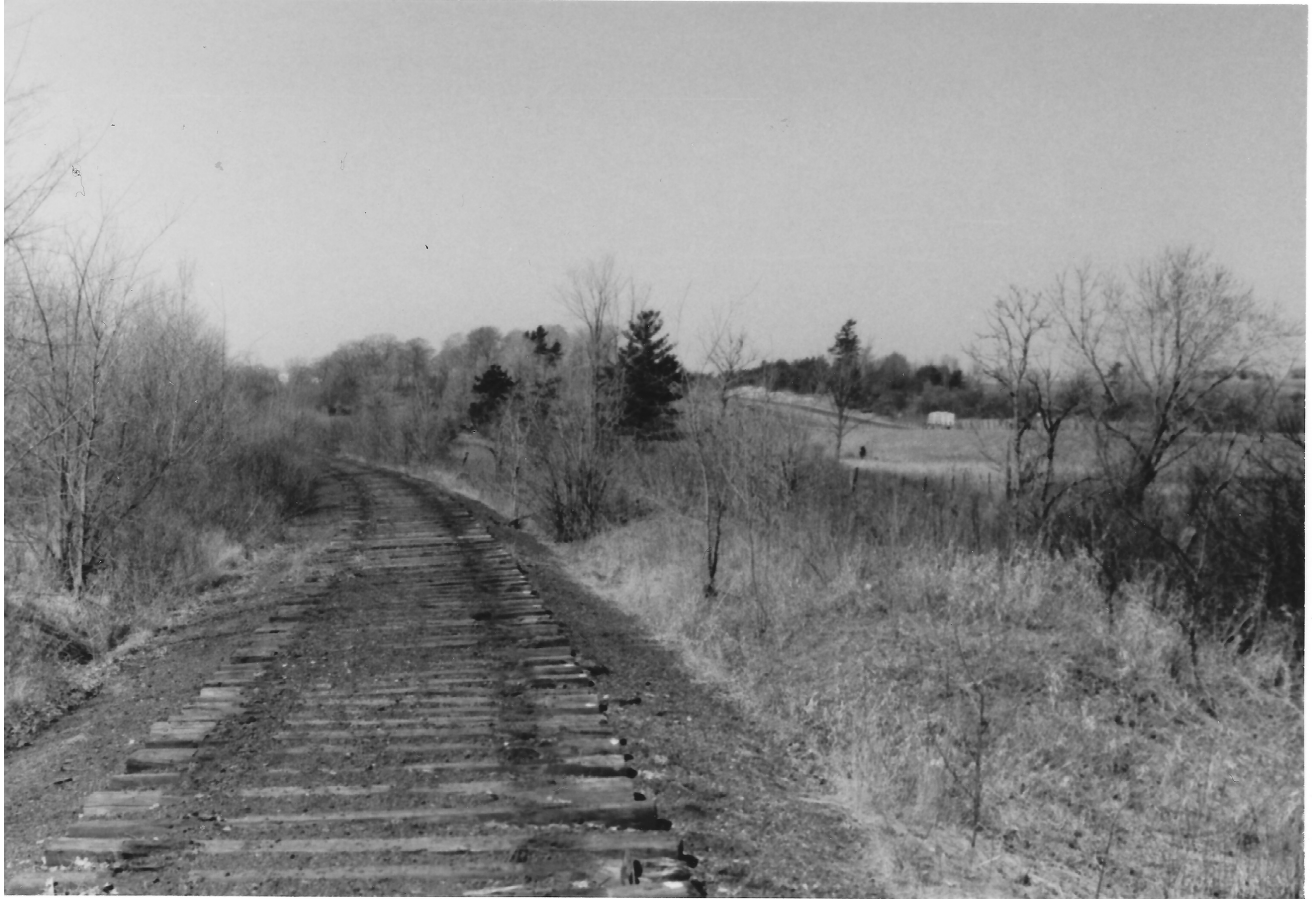
The rail line looking north from the Little Cataraqui Creek upgrade toward the Sydenham Road. The bridge over the creek is in the centre of the photo. The rails were lifted and hauled away during January. These ties were taken up during March 25 th and March 26 th .
