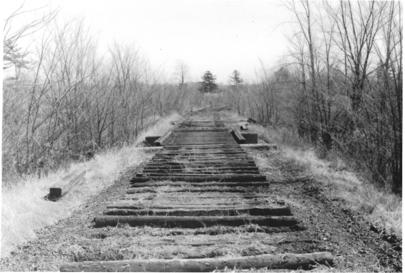
The rail line looking north upgrade at the Sydenham Road crossing. The old barn is at the left.
