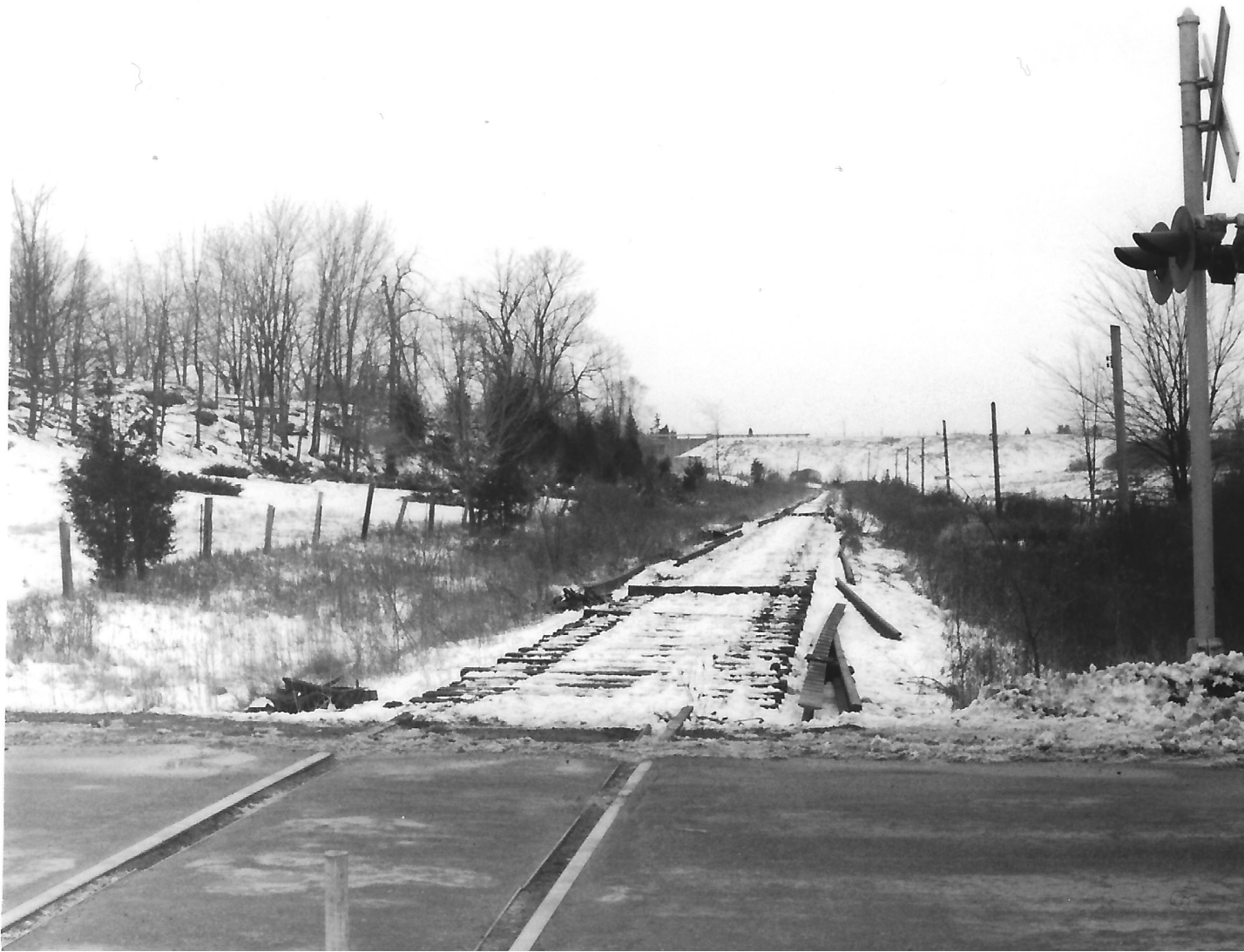
The rail line looking south from the Fifth Concession Rd. crossing at Jacksons Mills. The mill building is at the right. The west rail, at the right, was lifted from the ties on the following day. [January 7 th , 1987]
