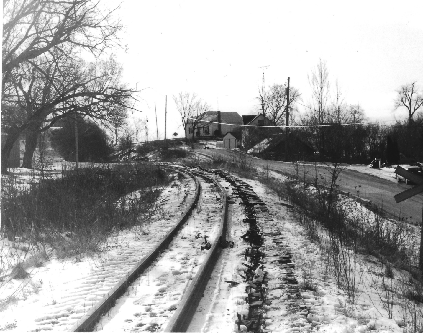
The rail line looking north at Jacksons Mills. The road crossing in the foreground goes into the home of Marvin Busch. The photo was taken one day after the west (left) rail had been lifted. Some of the lifted rails are lying over the on east rail.
