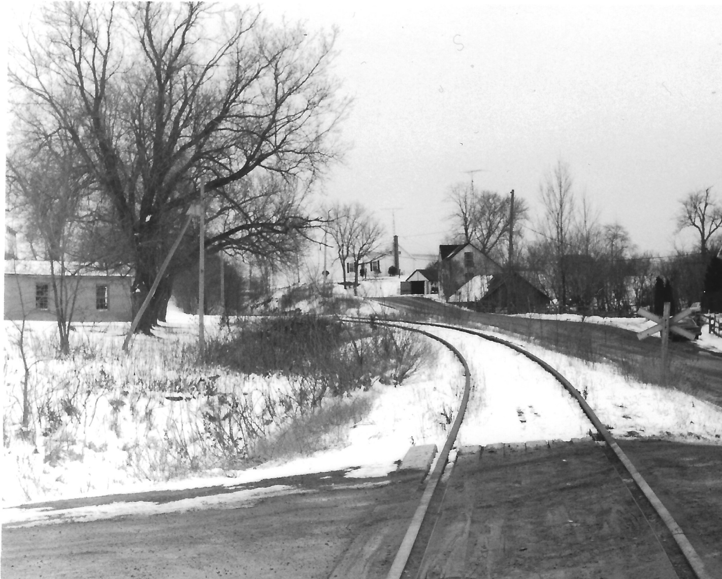
The rail line looking south to the rock cut at Jacksons Mills. The road crossing goes in to the home of Marvin Busch (formerly George MacRow). The farm home of George MacRow is at the top right. The west rail, on the right was lifted from the ties the next day [January 7 th , 1987].
