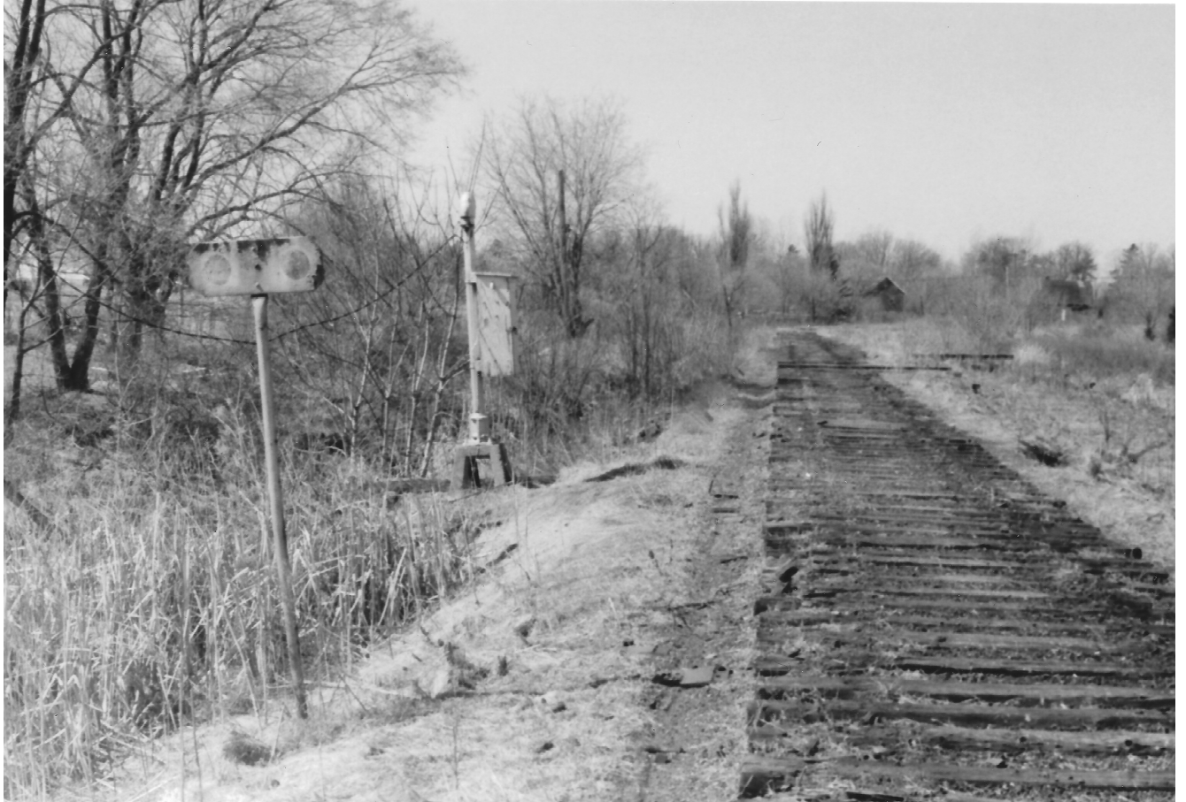
The rail line looking north upgrade toward the Sydenham crossing. The whistle board is for north bound trains approaching the road crossings. The rails were lifted and hauled away during January. These ties were taken up during March 25 th and March 26 th .
