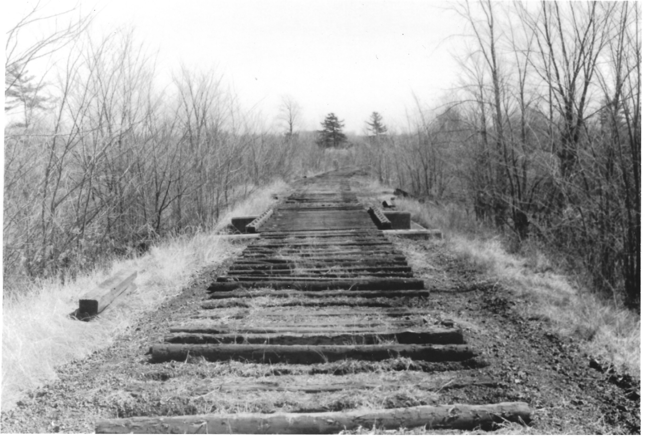
The K&P line at the bridge over the Little Cataraqui Creek, looking south towards Kingston.
