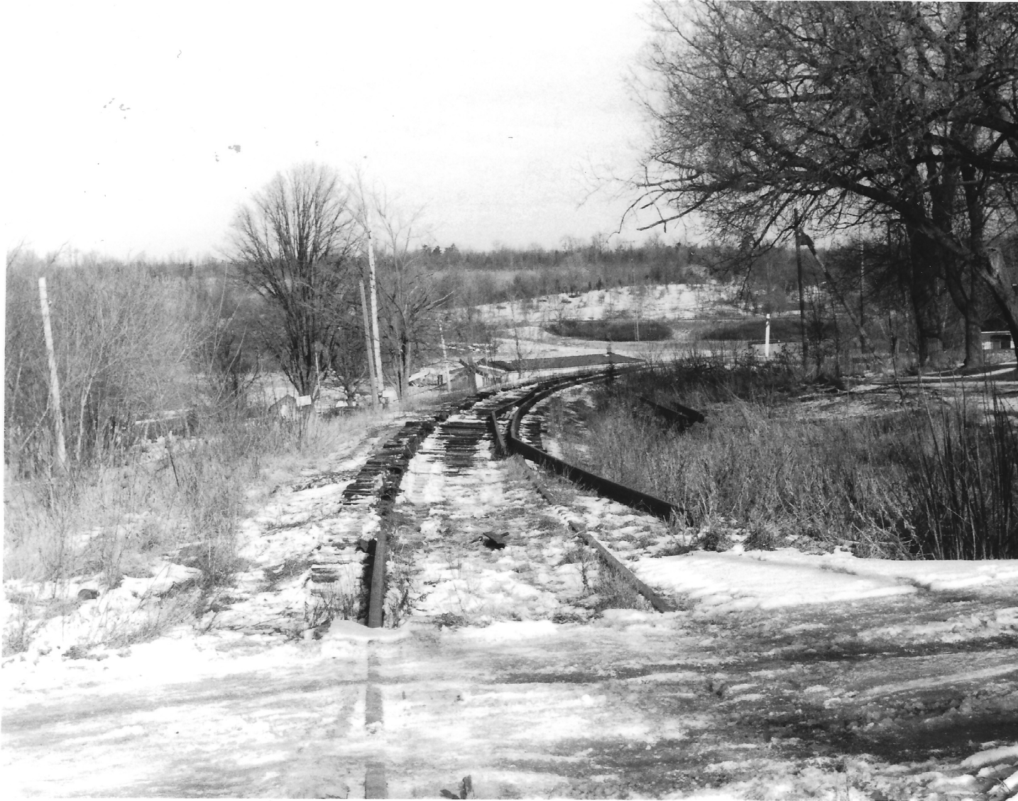
The rail line at the Cordukes Road crossing, looking south, at the intersection of the Fifth Concession Road. The former Jackson's Mills stone school house is at the right. The photo was taken one day after the west (left) rail had been lifted.
