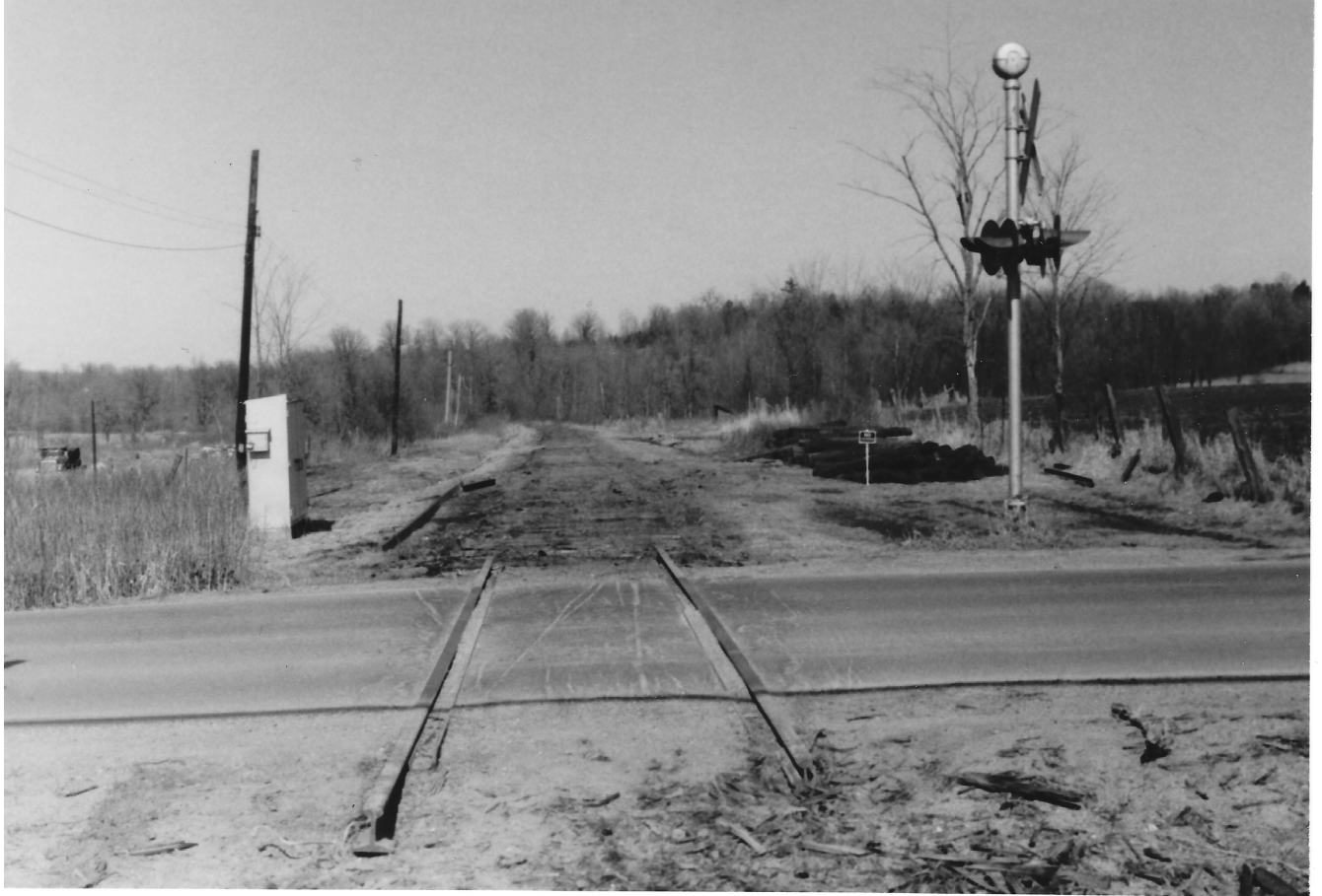
The rail line west of the McIvor Road crossing. Hwy 401 is in the distance. The rails were lifted and hauled away in January. The ties were taken up on April 10 th .
