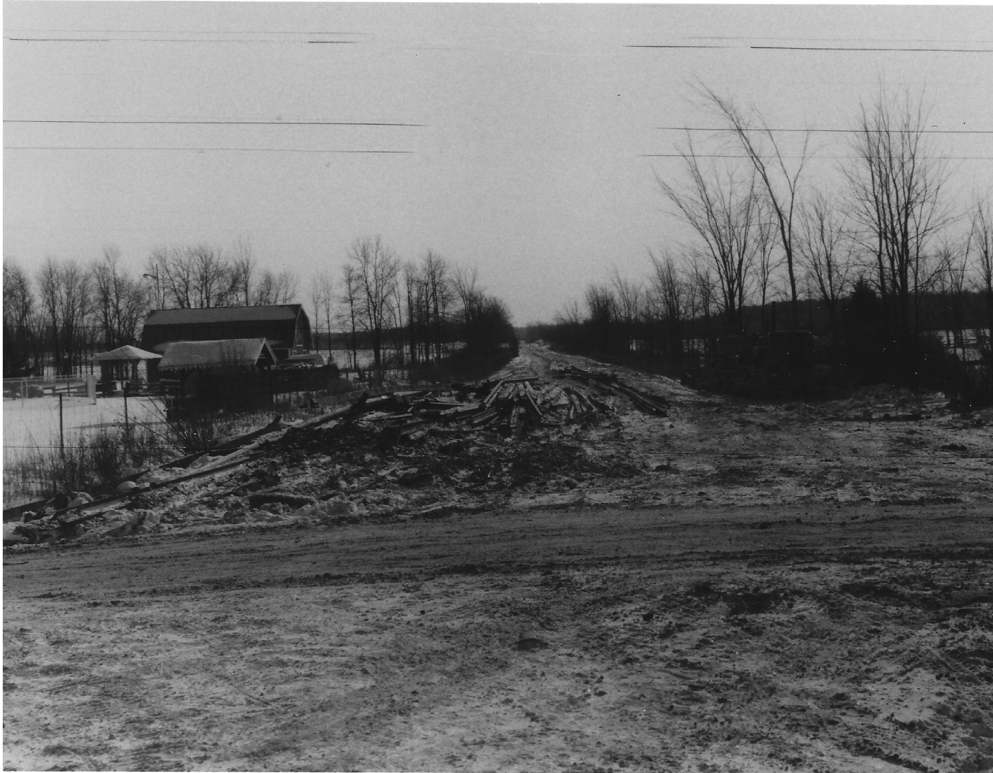
The rail line looking north from the Glenvale Station site. Elginburg Rd. crossing in the foreground. The rails have been hauled away but the ties are still in place.
