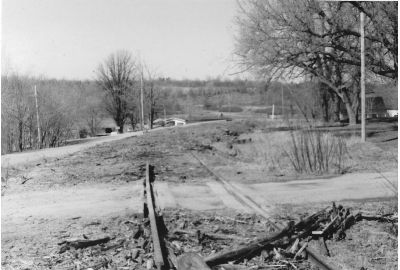
The rail line looking south from the rock cut through Jacksons Mills. Many of the ties were broken up by the bulldozers during the removal of the rail in January.
