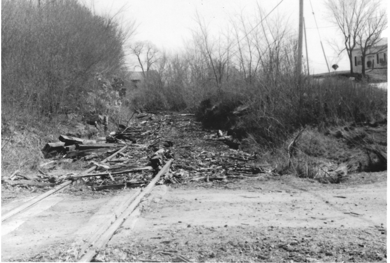
The rail line at the Glenvale Station site, looking south, from the Elginburg Road crossing. The switch lever post and wooden signal board of the north siding switch is partly buried in a pile of grass. The ties along this part of track were taken up and plied on April 10 th .
