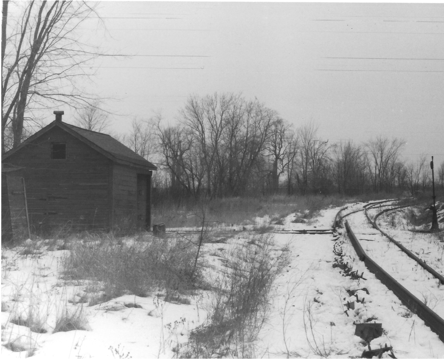
The rail line at Murvale Station site looking south. The west (left) rail has been lifted. At the right is the trolley shed. The siding swings in to the left from the south end switch.
