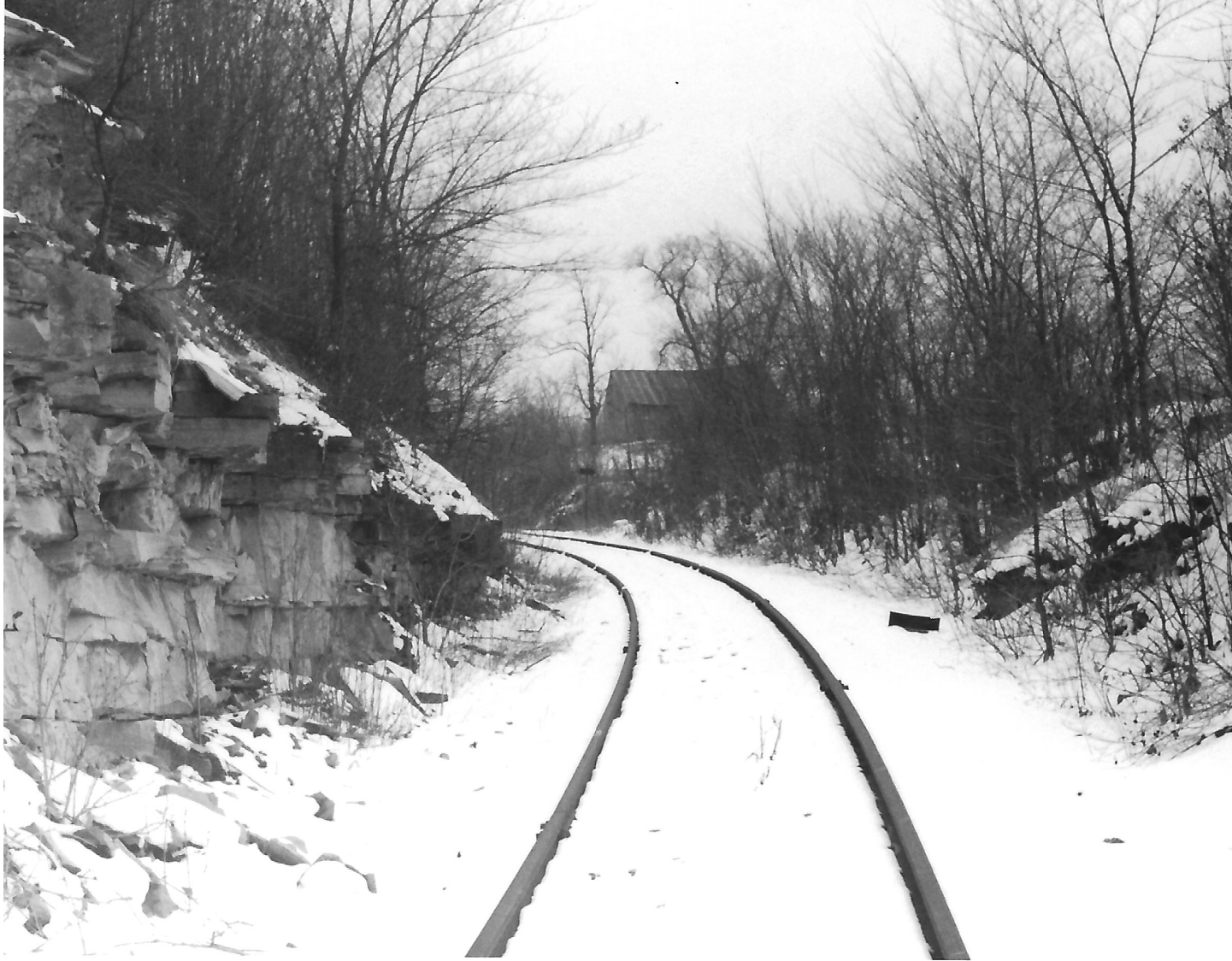
The rail line looking north from the Fifth Concession road crossing at Jacksons Mills. The track curved in to the large horseshoe bend, around to the left, and up the grade to Cordukes Road.
